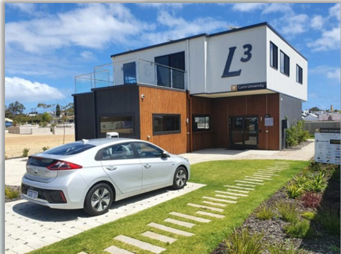
Figure 4 Legacy Living Lab Building (Curtin University, 2021)
